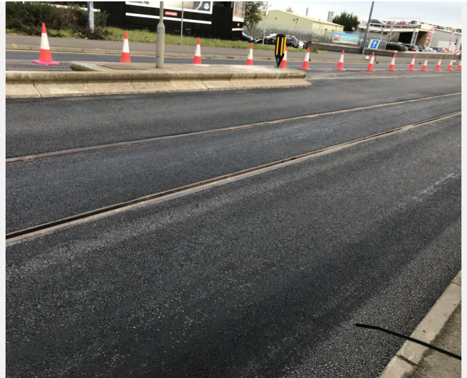
Secure embedded tram tracks
