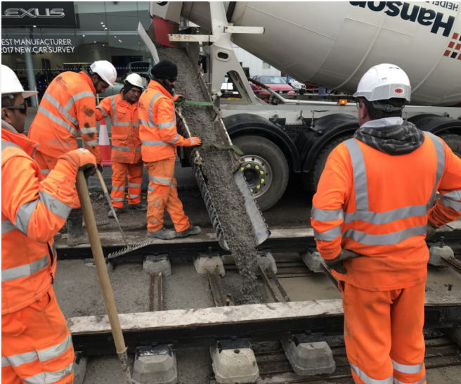
Concrete direct to the track base
