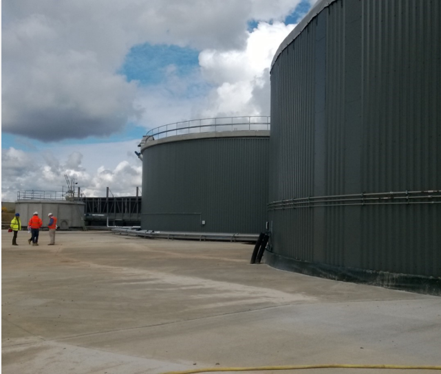
Large areas can be poured straight from the truck without the need for pumping.
