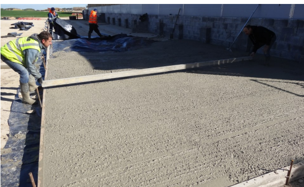
Durus EasyFinish C40 slump concrete for a pig farm sump base.
