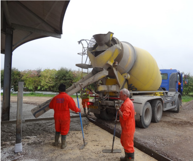
Concrete discharged directly into the shuttering
