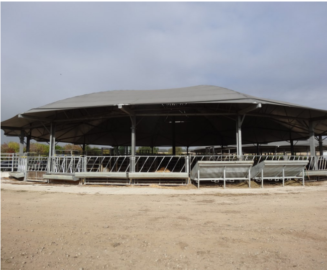
Shed in use sooner, due to quicker installation
