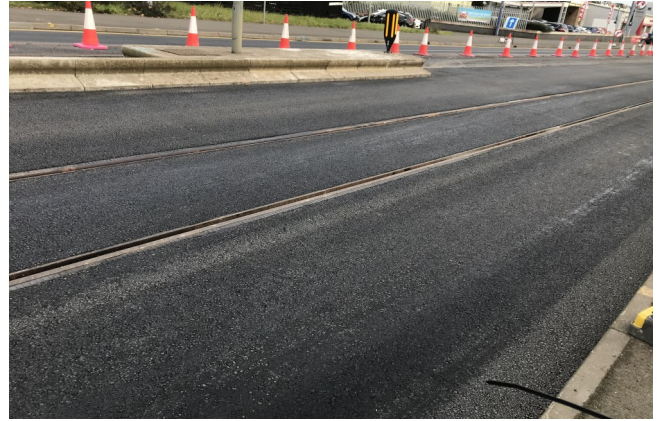
Secure embedded tram tracks
