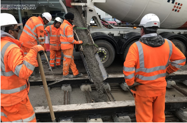
Concrete direct to the track base
