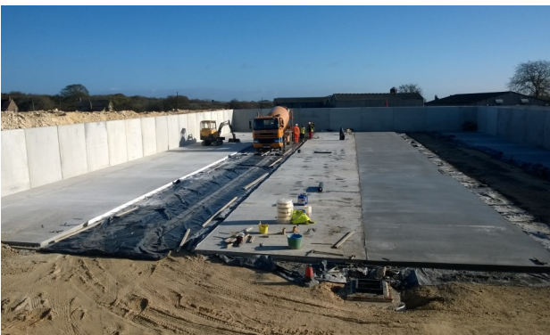
Durus C40 slump concrete for silage clamp base.
