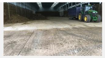
With the elimination conventional Steel Mesh, large strips pours can be completed, allowing quicker construction.
